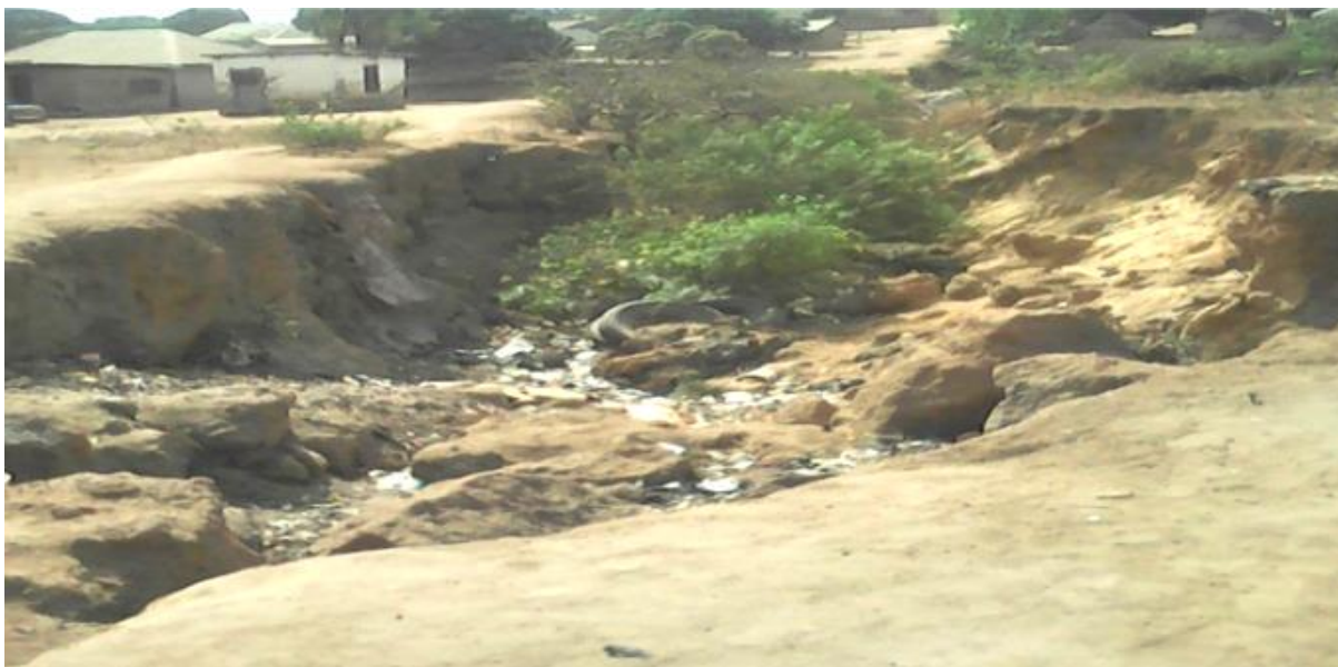
Plate 1: A typical gully head in a built-up area (St. Thomas Primary School) in Gboko: Note: The gully wall recession and presence of waste materials in the gully channel. Photo by: The Authors, January, 2017.
